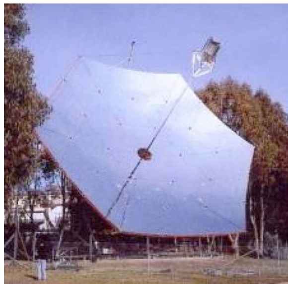
Fig. 9. The SG3 Big Dish prototype was built in Australia in 1994 and is the world's largest solar dish for generating electrical power, with an average diameter of roughly 23 m. It achieves a solar concentration of 1500 suns, and heats water in the range 400^\circ\text{C} – 700^\circ\text{C} at 4.2–6.8 MPa. It has a design output of 320 kW. Source: Australian National University (ANU).
