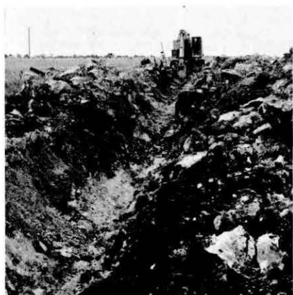
Excavating blasted rock.
