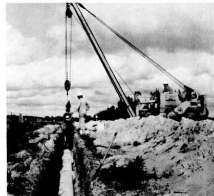
Laying 10 in. Fibrolite AC pipes with a pipelayer.
