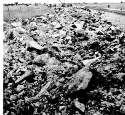
Line of a branch main after blasting.
